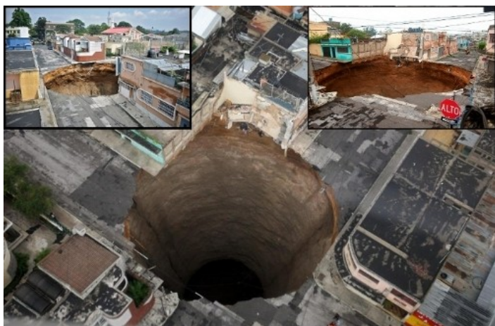
Guatemala City sinkhole - May 31st 2010
